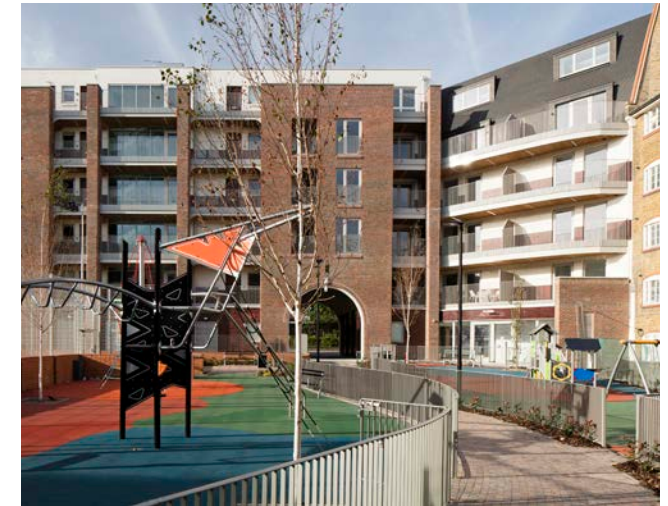
Estate regeneration including new mixed tenure homes, a community centre and a Multi-Use Games Area for social and physical well-being. Bourne Estate, Holborn, London.
