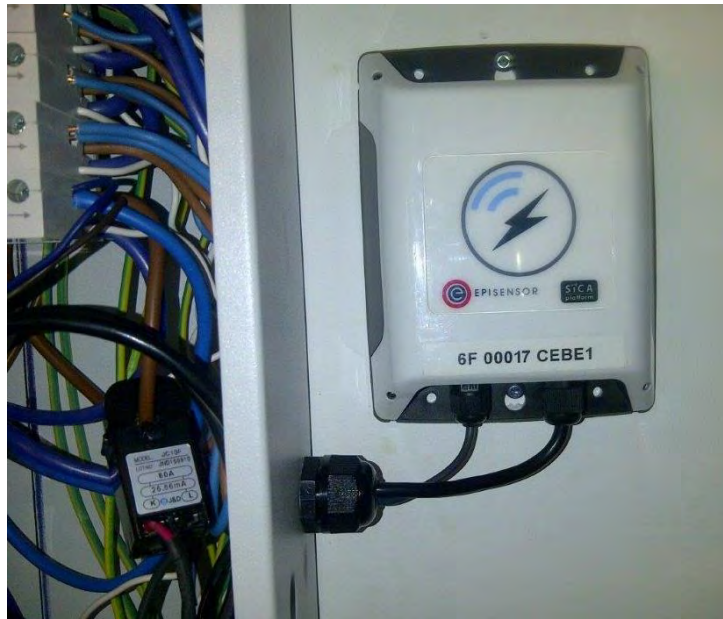
Figure B 10 – ZEM-30 single-phase monitor with current transformer
