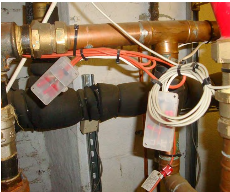
Figure 66 – Temperature sensor leads extended
