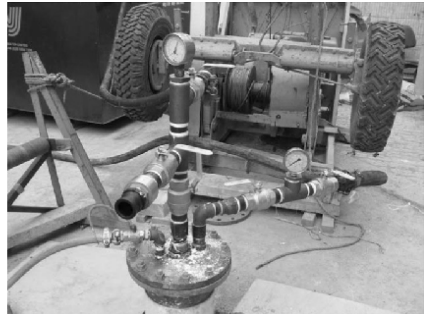
Acidising well to increase flow rate
