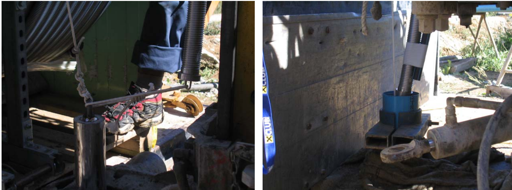
Source: Insertion of the CO 2 -tube (Ochsner GmbH)
