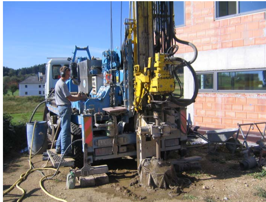
Source: Drilling of the borehole (Ochsner GmbH)
