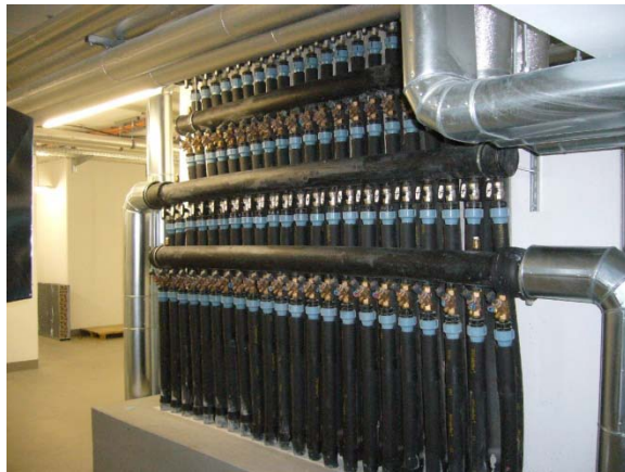
Heat pump and BHE manifold for county administration Gelnhausen (86 BHE)
