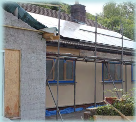
External insulation on the building
