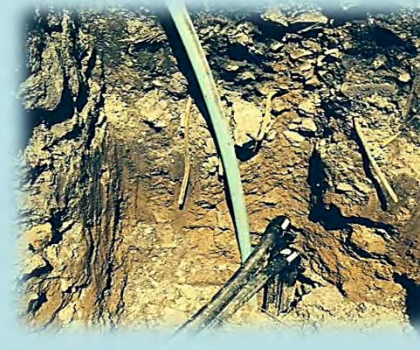
Typical vertical borehole
