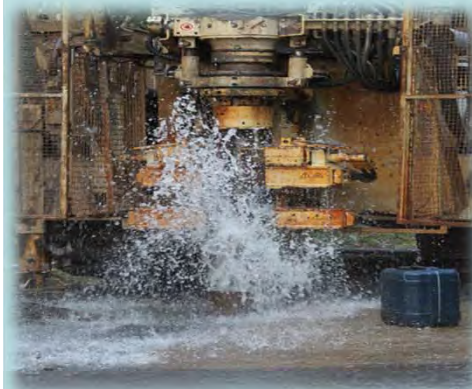
Drilling in action
