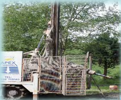
Drilling in progress
