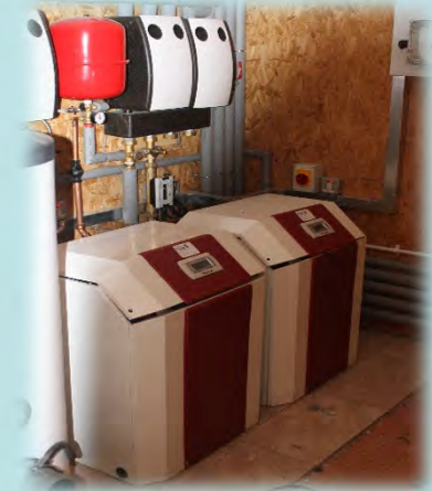
View from Plant Room
