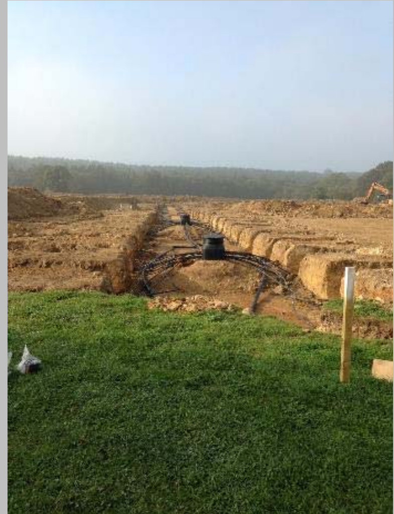
Construction of the chamber
