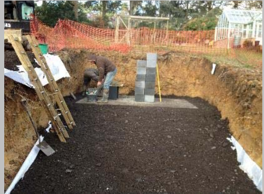
Construction of the chamber
