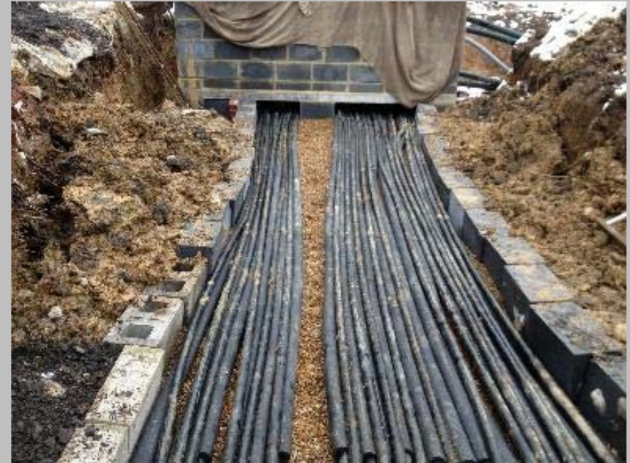
Flow and returns to collector
