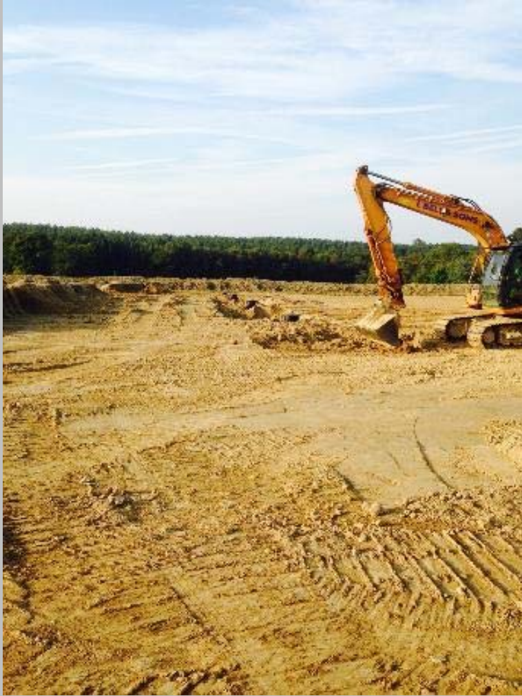
Careful backfilling around manifolds
