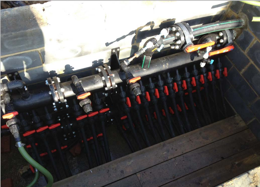
Central Manifold manufactured by Baystar
