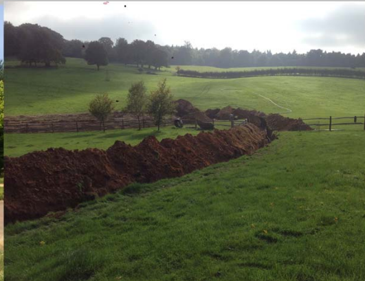
Trenches for coils
