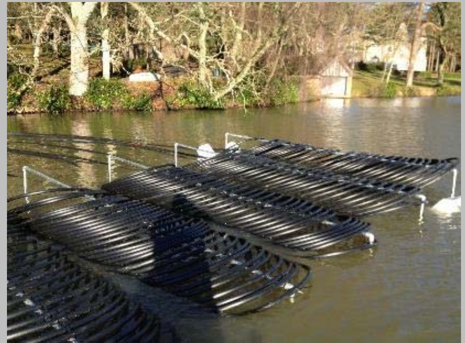
Float on to lake and bolt together
