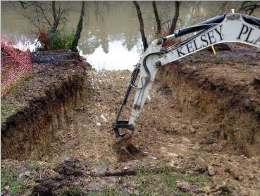
Installation starts at the manifold
