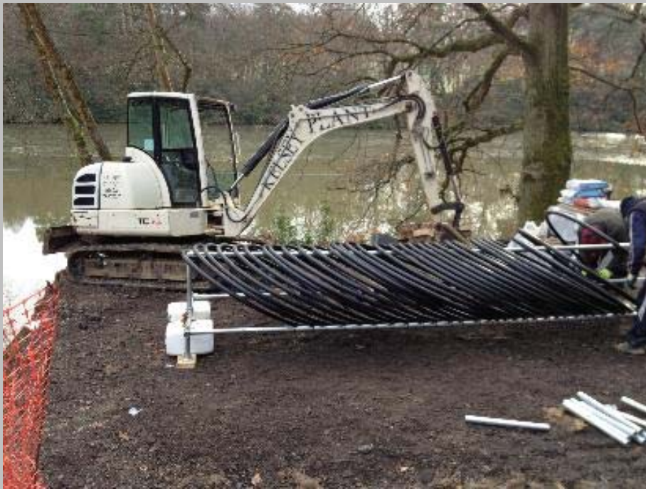
Collector loop construction
