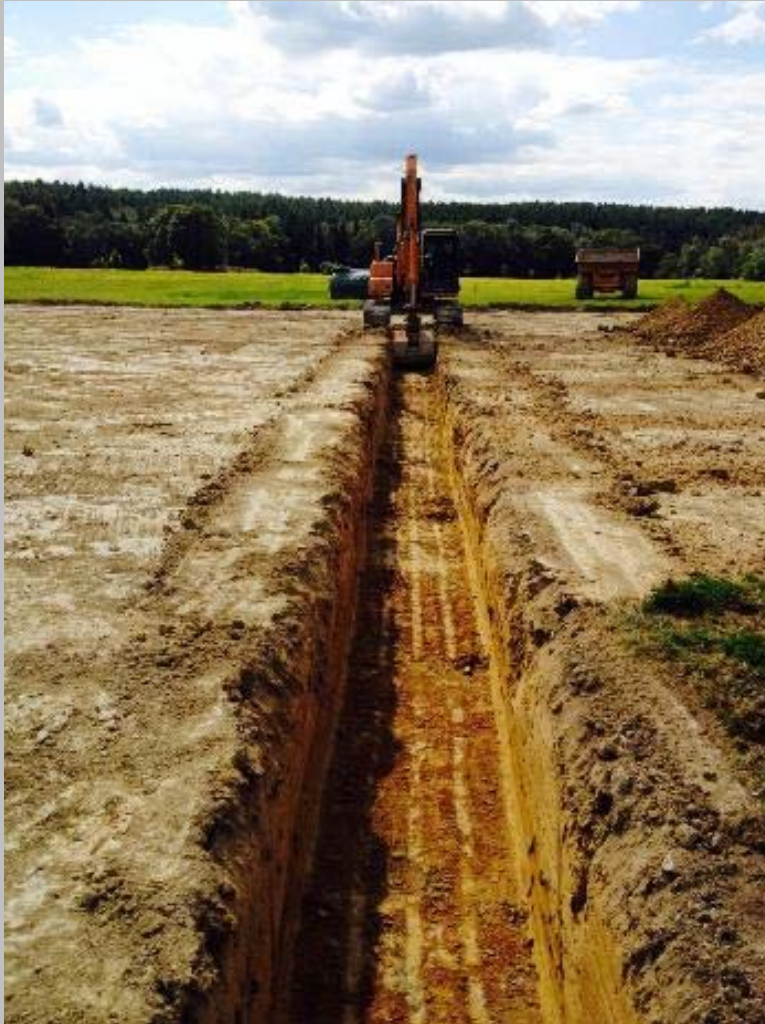
Installation starts at the manifolds
