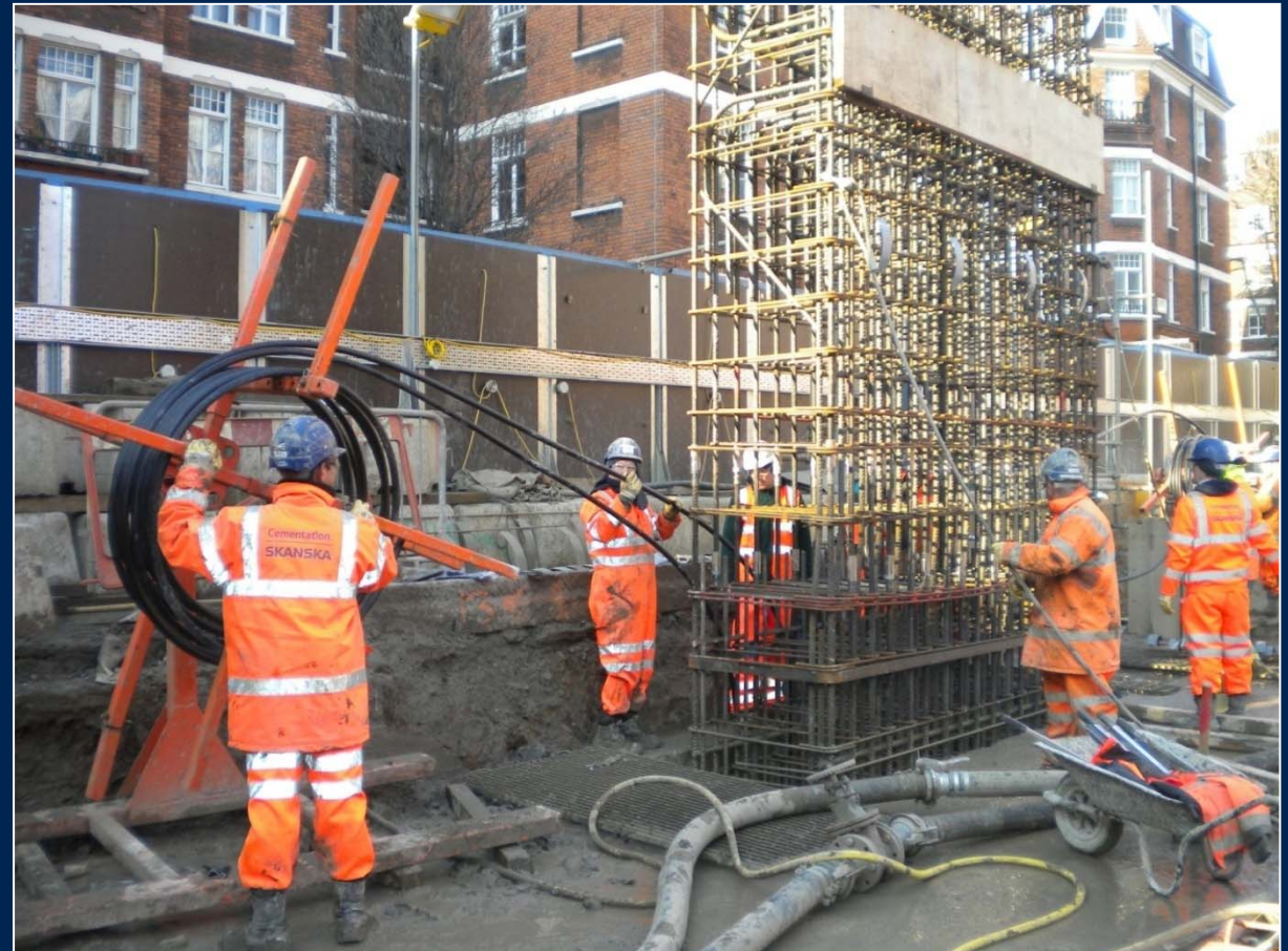
Thermal loops prefixed on inside of reinforcement
