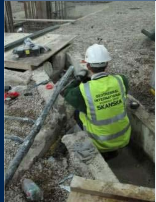
Clash with headering and drainage
