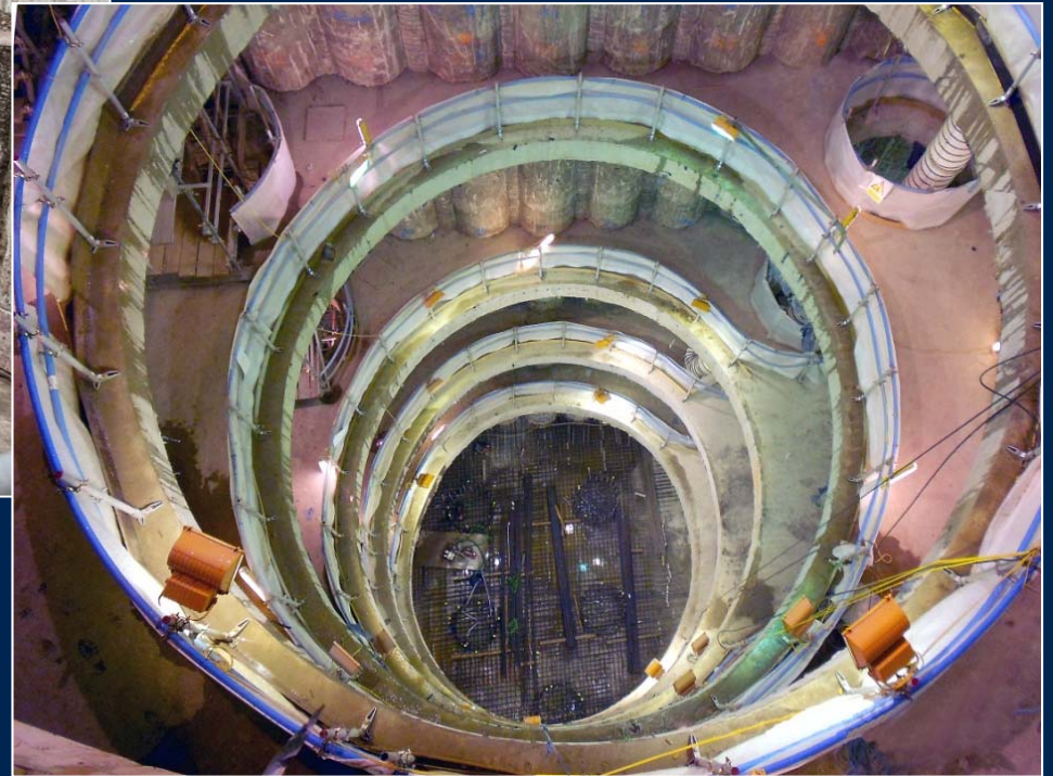
Thermal piles at base of shaft
