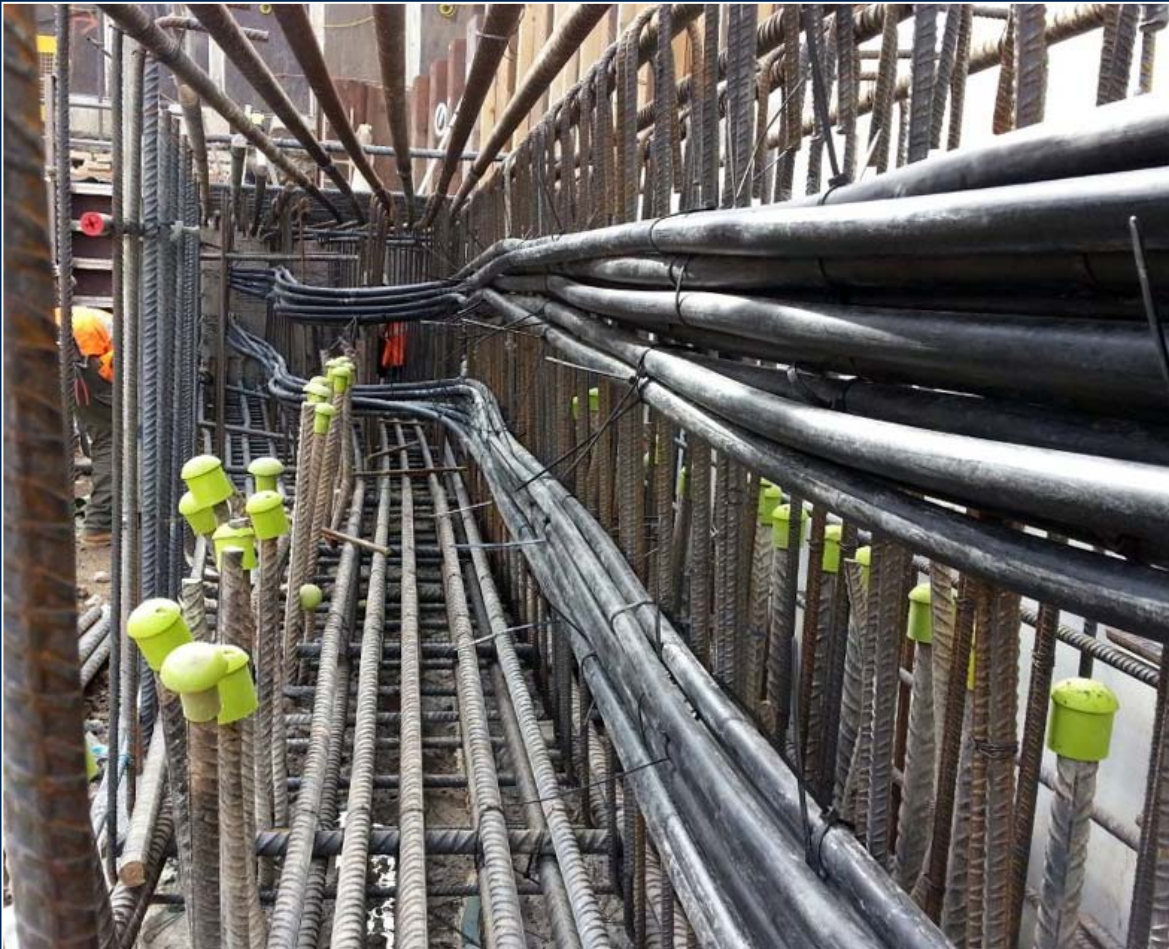
Loops collecting up inside the capping beam
