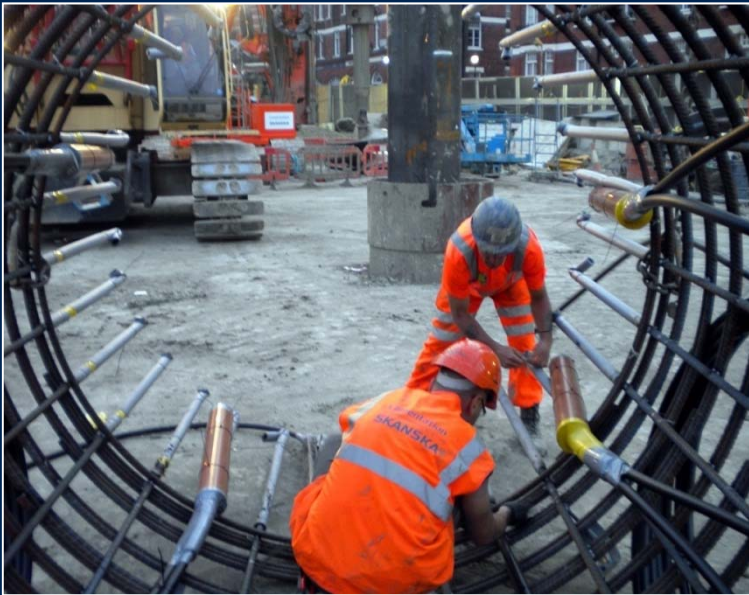
Thermal loops prefixed on inside of reinforcement
