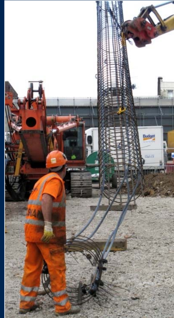
Loops fixed on inside and extend below the cage using a cage former
