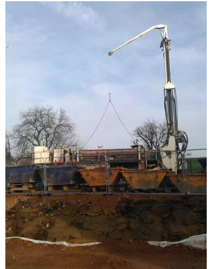
Lifting casing into place
