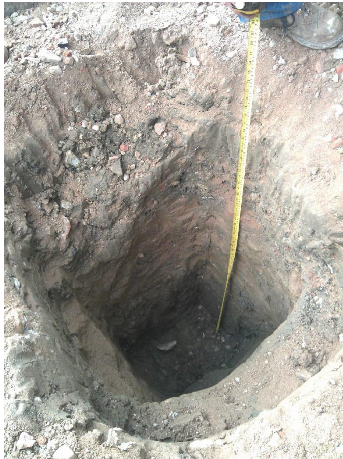
Hand dug pilot hole
