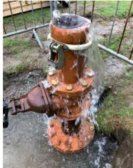
Temporary wellhead on artesian borehole
